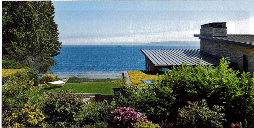
By anchoring Manlowe's lower home into the hillside and installing a green roof system, the roof form blends into the landscape, Coates says, and does not compromise the view from Bryant's home.
